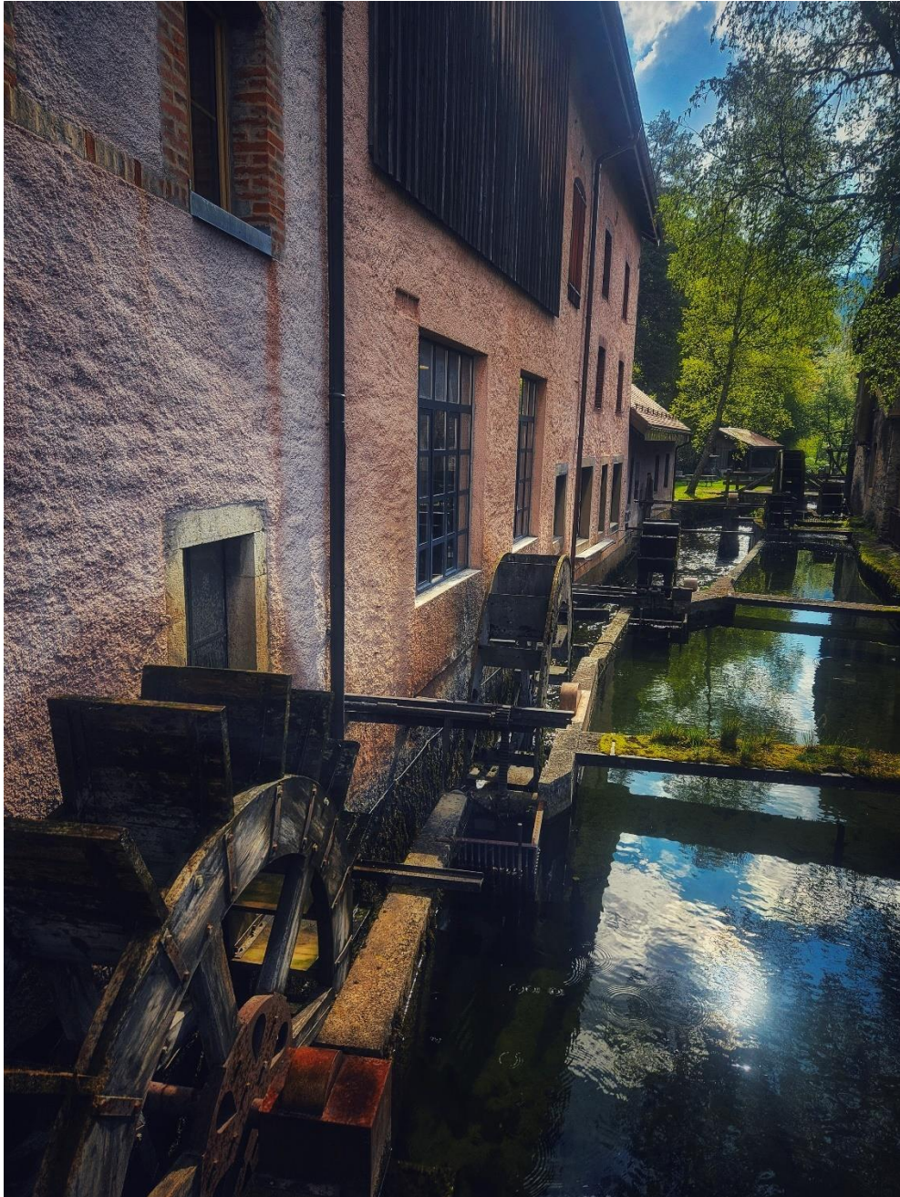
View of the branched canal of the Orbe and the mounted water wheels
